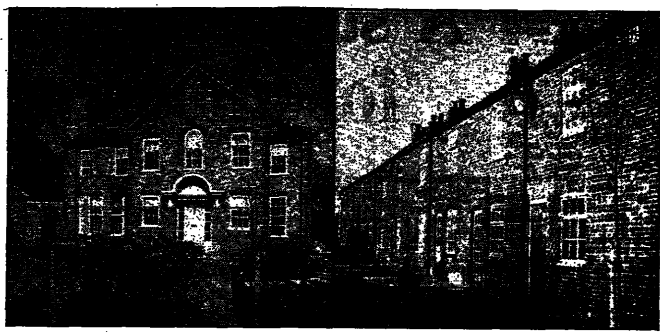
Above: Barratt's neo-Georgian Dulwich Gate estate, with prices between £400,000 and £500,000. The development, to comprise 23 houses, has won a number of awards for its high quality. Right: Black Road, Macclesfield, where the pioneering idea of community-based regeneration was born in the early 1970s, is still a symbol for the kind of achievement possible for many inner-city communities.
